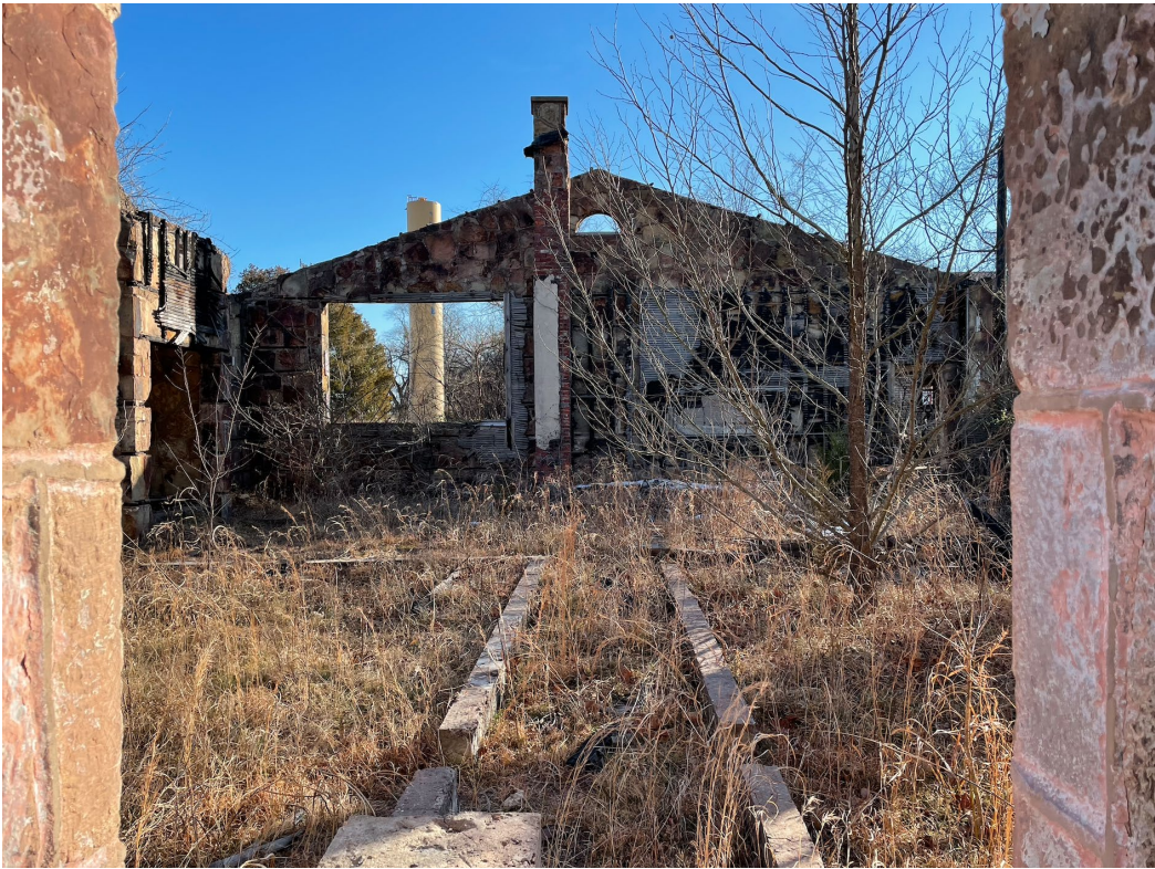
Figure 3 - Interior view of existing south section of building, facing south.
